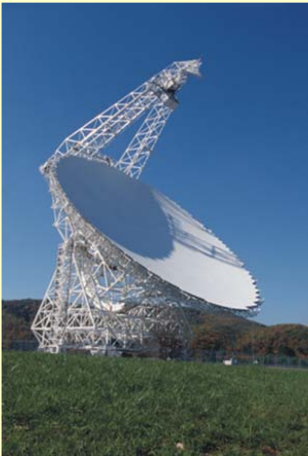
Green Bank 100m Antenna
