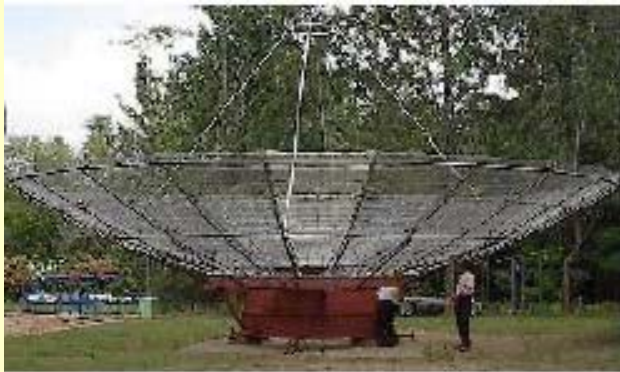
PDD - a 12 meter Preloaded Parabolic Dish
